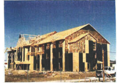
Framing lumber, floor, wall and roof sheathing plywood
